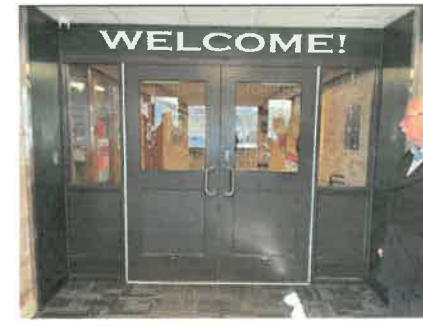
REPLACEMENT - THIS IS AN EXTERIOR ENTRANCE DOOR THAT WAS RECENTLY REPLACED, THAT THEY WANT TO MATCH
